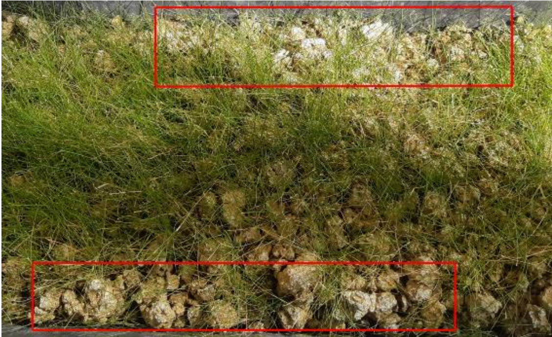
Figure 5. 17. Presence of salts on sediments surface
