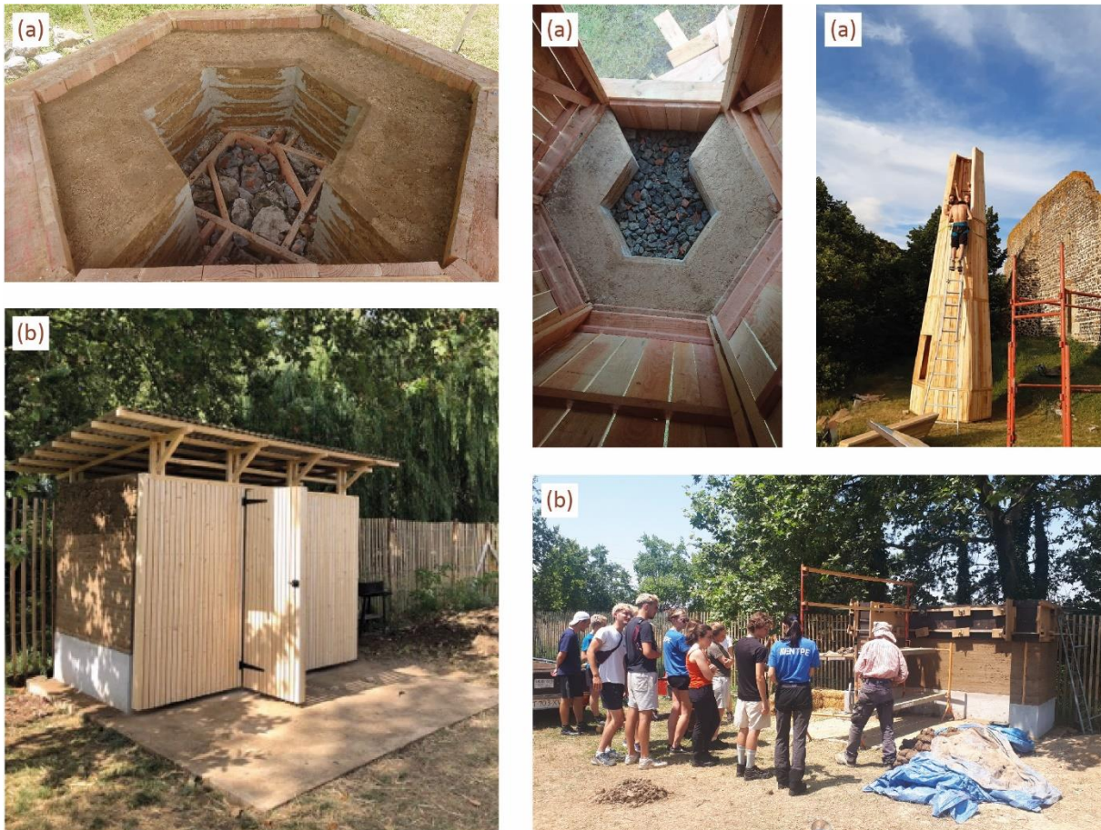
Figure 0.19: (a) Construction of a place of meditation on the pilgrimage route to Santiago de Compostela, Montverdun priory, base made with rammed earth and wood structure, the construction was temporary and meant to stand for a year (source: author); (b) Construction with ENTPE students of a garden sheds for inhabitants (source: author)
