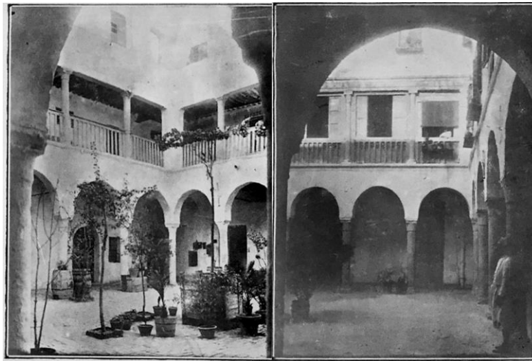
Figure 36. Patio du palais (Source: Grandchamps, 1932)
