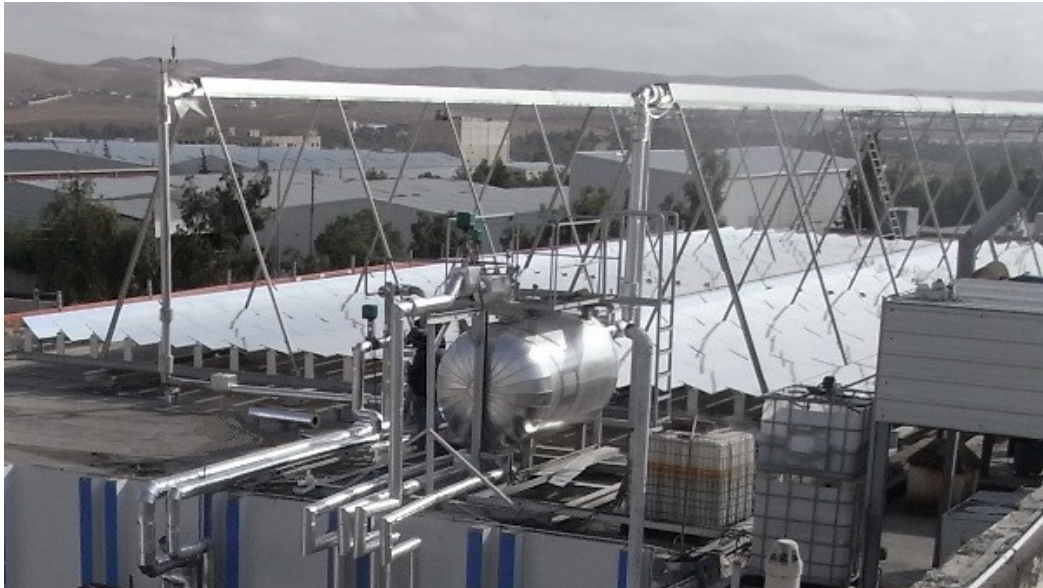
Fig. 1.6 LF-11 Linear Fresnel Collectors built by the company Industrial Solar at RAM Pharma, Amman (Jordan). Source: DLR Institute of Solar Research website 4
