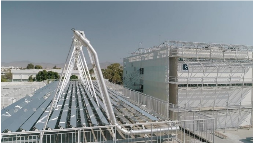
Fig. 1.7 Linear Fresnel Collectors installed at the Cyprus Institute (CyI). Source: Cyprus Institute (CyI) website 5
